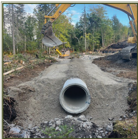
Port Hawkesbury Paper watercourse crossing construction
