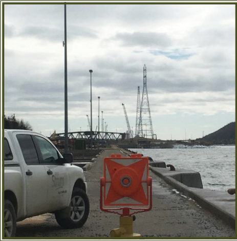
Strait of Canso Causeway transmission line and towers topographic survey
