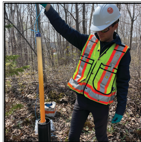
Groundwater well installation and monitoring at Burnside Composting facility
