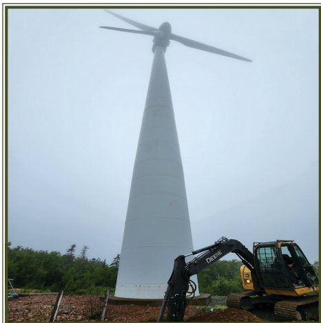
Higgins Mountain wind farm construction monitoring - post EA approval
