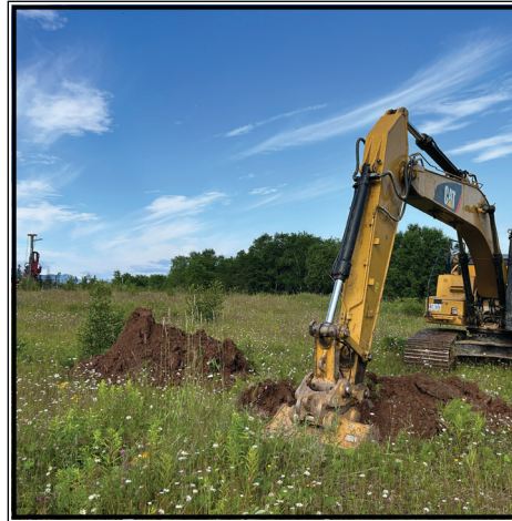
Test pit investigation to collect subsurface samples for a proposed new building development
