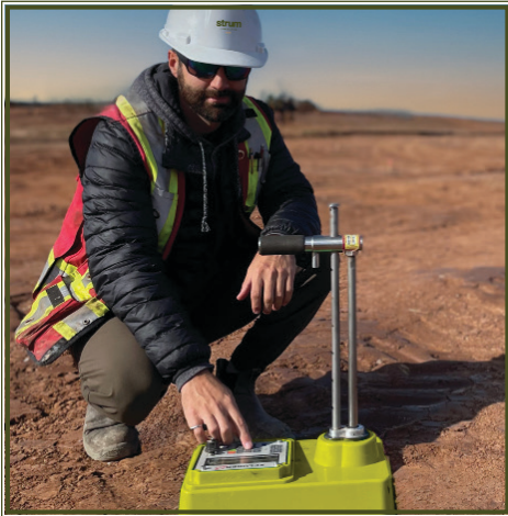
Soil compaction testing during cut and fill operations
