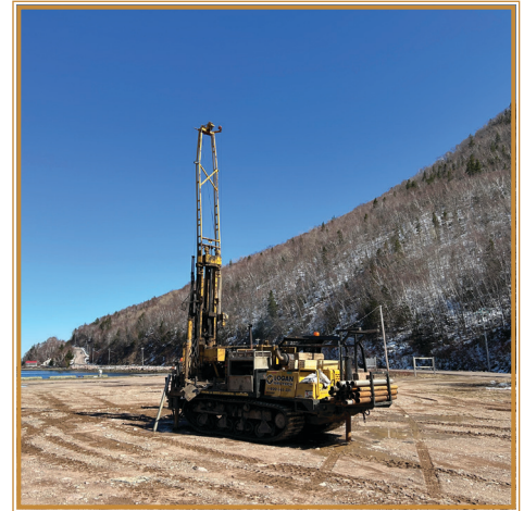
Borehole field program to obtain bedrock depths to support civil design
